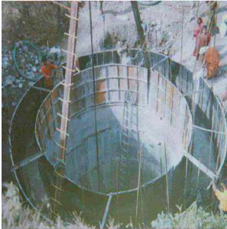
SHUTTERING WORK IN PROGRESS WELL FOUNDATION OF SIMBLE Br AT KM 18.0 ON SIMBLE Br JAMMU-AKHNDOR ROAD
