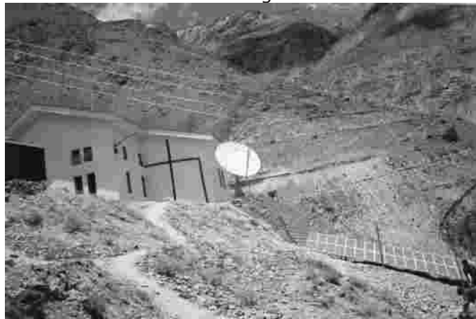
Figure 6.57 SPV for satellite earth station
