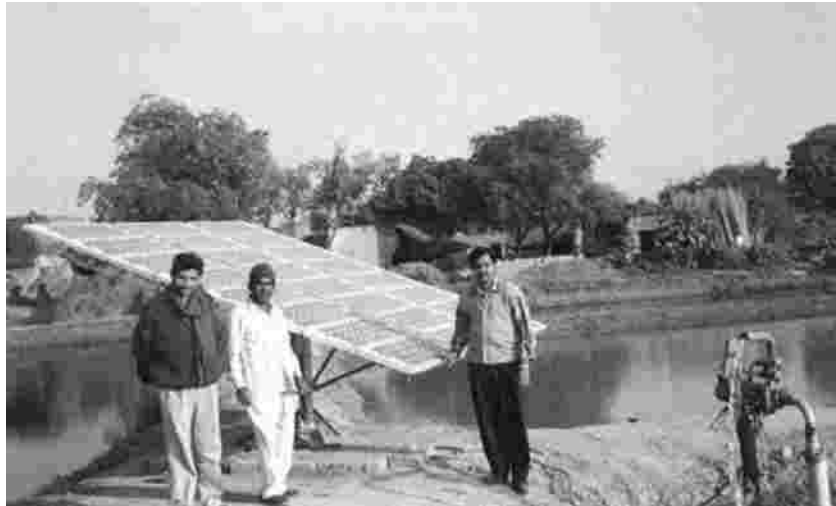
Figure 6.53 An SPV water pumping system for fishing farm
