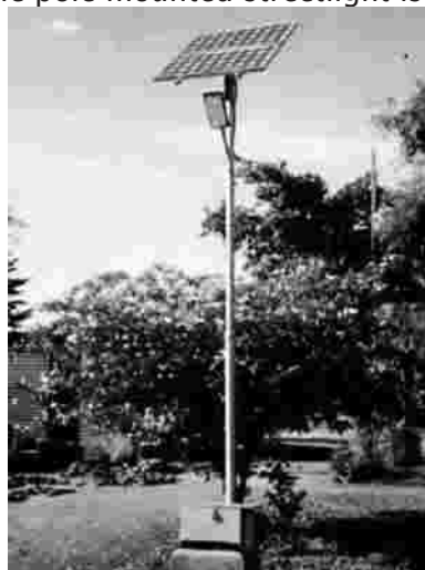
Figure 6.54 Pole mounted SPV lighting
